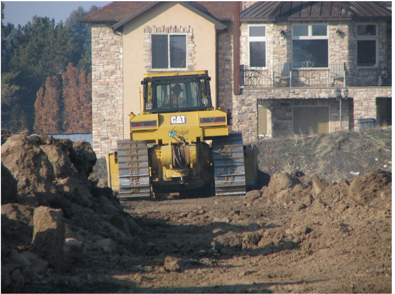
Looking west at the dozer pushing waste towards the working face
